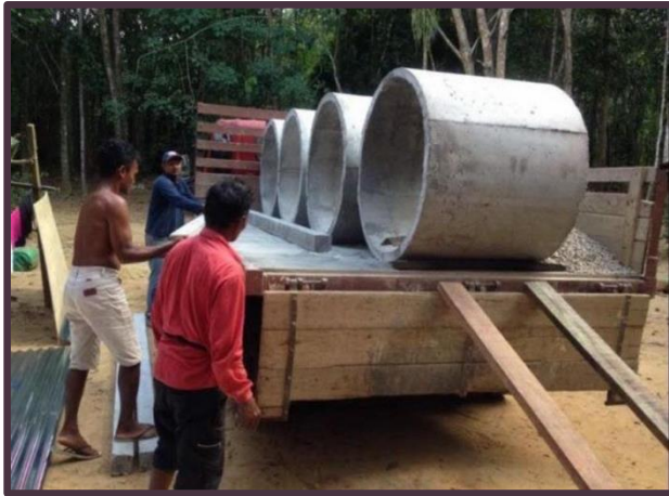
(L) Each well has 3 cement rings and a water pump using petrol or generator is given with a 600 gallon tank and tap water is produced
