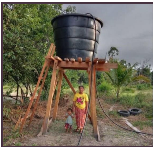
(L) A 600-gallon water tank is given for each well and with the pump, tap water is produced (R)
